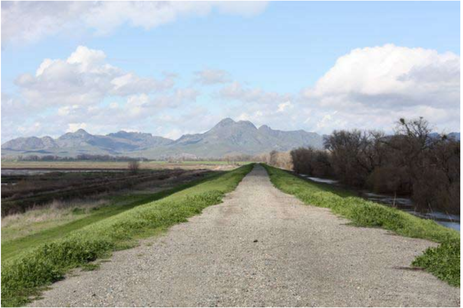
A graveled road atop the east bank levee of the Sutter Bypass, looking north toward the Sutter Buttes. Sutter County has 240 miles of levees.
