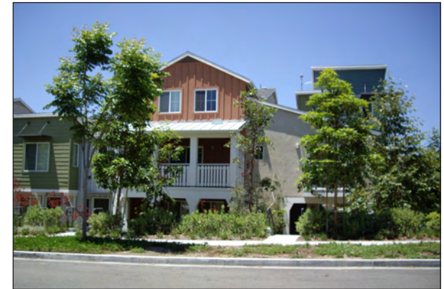
Tree planting should be used to soften the visual mass of buildings.
