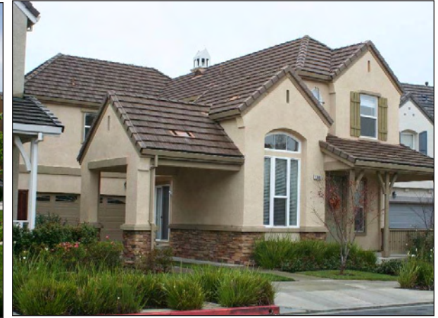
Recessed garages to rear of lot accessed from local street
