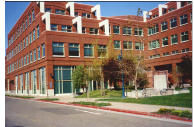
Massing of three-dimensional volumetric forms of large industrial buildings should be broken into smaller components, where feasible.
