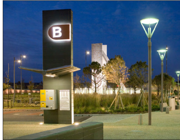
Parking lot lighting should be no higher than necessary to provide efficient lighting of the area.
