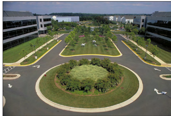
Organizing business and industrial park buildings along a major circulation spine is encouraged.
