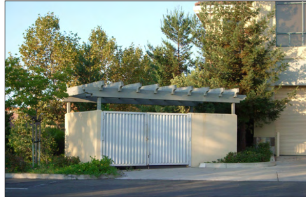
Trash/recycling areas within commercial and multi-family residential areas should be screened by minimum 6 foot-high walls and/or landscaping.
