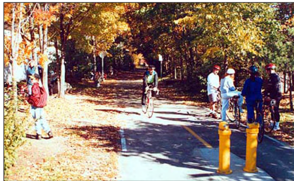
Off street bike-paths and pedestrian trails should discourage inappropriate vehicular use by providing vehicular barriers, such as bollards.
