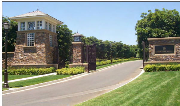
Community gateways and entries should be designed to establish a sense of place and reinforce a distinct character for the community.
