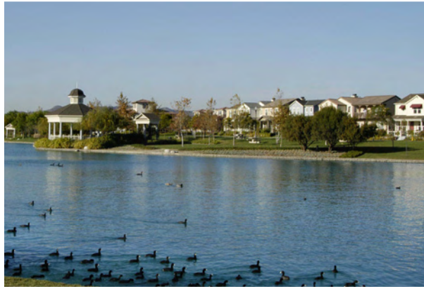
Residential villages are organized around parks, open space amenities and drainage features.
