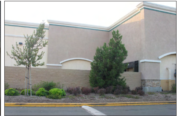
Loading and trash areas should be located behind or at the side of buildings and screened with walls and landscape planting.
