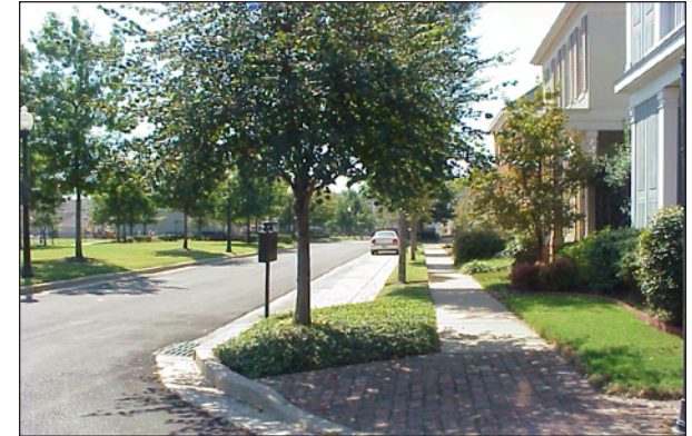
Canopy trees in landscaped parkways and on-street parking with bulb-outs at intersections along local streets provide a safe and comfortable environment for pedestrians.
